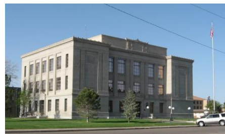
Prowers County Courthouse
